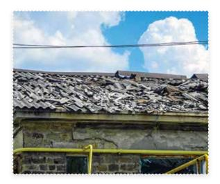
According to information of the Healthcare Department of Luhansk Oblast Administration, a total of 15 windows and 145 glass units, 90 meters of gas pipes was damaged; the shell broke through 16 m2 of the wall 1,419 m2 of roof slates, and 48 m2 of partition walls.
